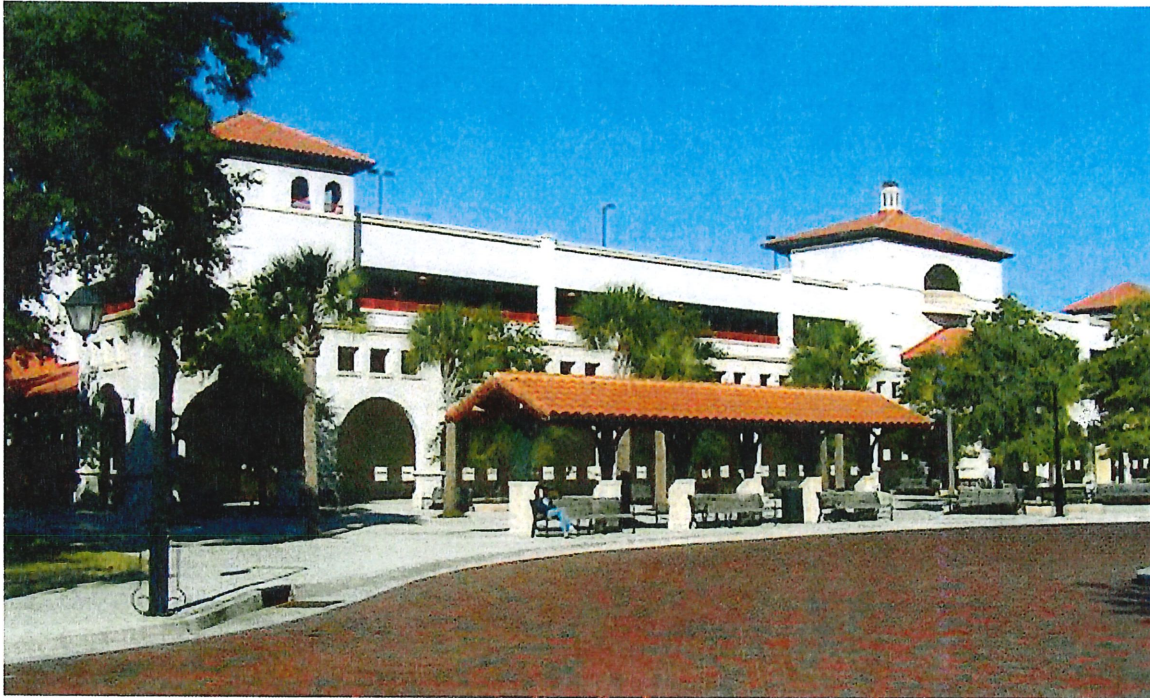
Figure 11. Historic Downtown Parking Facility (Garage)
