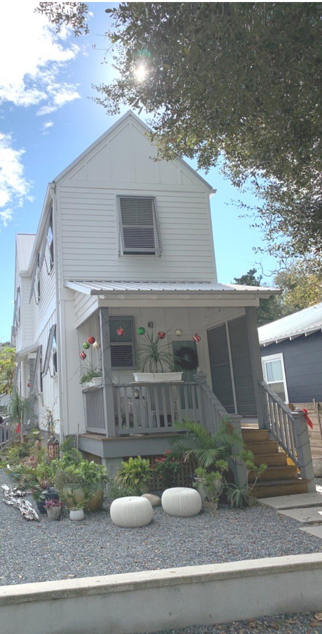
A low site wall can help to provide flood protection. Also shown is an open "pier system" for the front porch.
