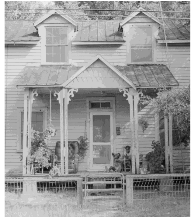
Metal and wood fencing. Image from Florida SP Lincolnvile Historic District document.
